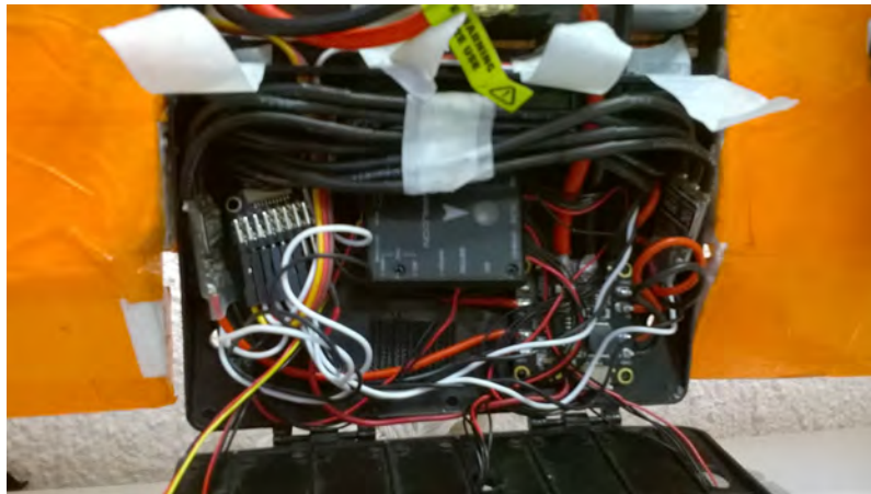
(a) Internal fly control system
